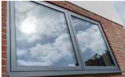
WAF ALUMINIUM FRAMED WINDOW ASSEMBLY POWDERCOAT FINISH IN COLOUR 1
